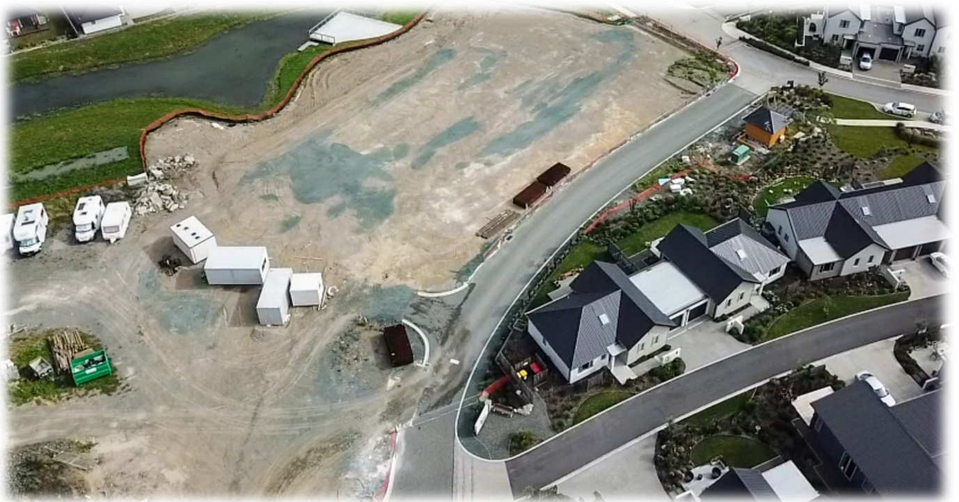
Aerial of the Lakehouse Build Pad
